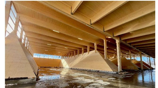
For the salt warehouse, We Construction and Cinis Fertilizer have chosen to construct the frame, roof and salt partitions in cross-laminated timber, as this creates significant sustainability gains. If the partitions in the salt warehouse had been constructed using concrete instead, this would have necessitated large quantities of reinforced concrete in order to withstand the substantial unilateral pressure created by 10 m<sup>3</sup> of salt.
