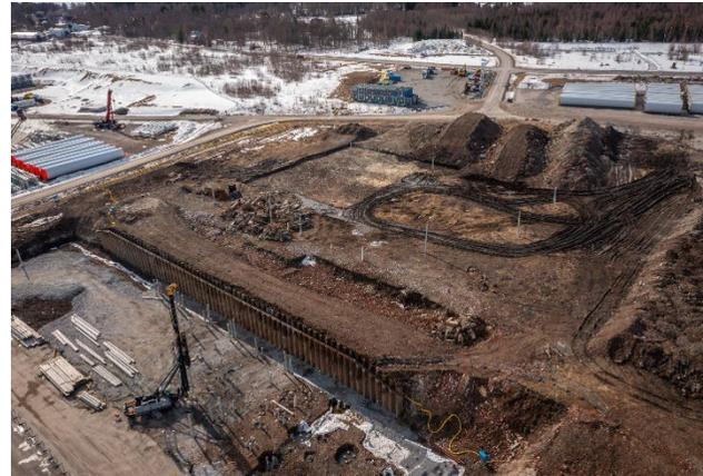
A large part of the site has been decontaminated following a decision by the County Administrative Board, and soil and rubble that falls below permitted levels has been reused on site as a noise barrier. During the decontamination process, construction rubble has been separated out and reused on site. Approximately 700,000 kg of residual concrete has been reused, alongside 110,000 kg of scrap steel which was removed from the site and sent for recycling.
